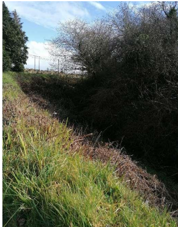
Outer slope of embankment with moate above.
