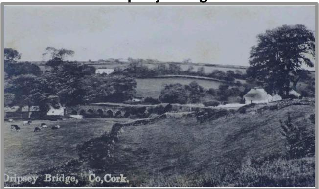
Dripsey Bridge is shown on the 1811 Grand current bridge has six semi-circular arches Jury Map of the area and was initially a small with three overflow arches at the eastern stone structure. bridges, it was possibly enlarged upon by to support the centring of arches during local landlords and magistrates (local Grand construction. The riverbed is paved beneath Jury) through Westminster funding in the the early 1820's It is reputed
